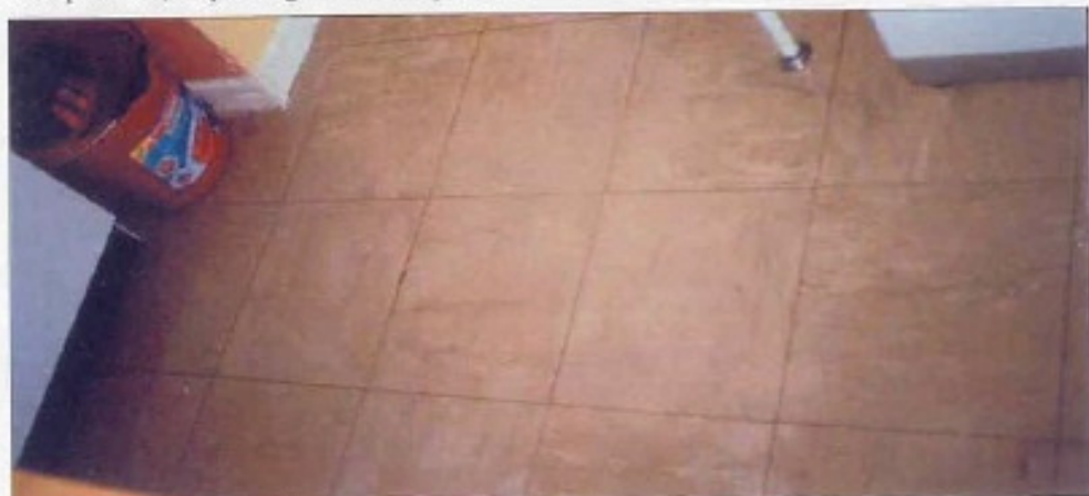
Floor tiles cleaned using Safe Paint & Varnish Remover.
